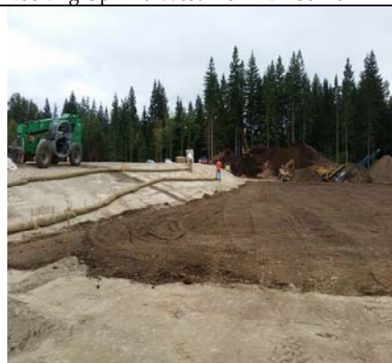
Installing Erosion Control Hay "Waddles"
