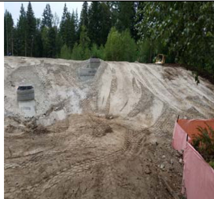
Looking Up And West From NE Corner
