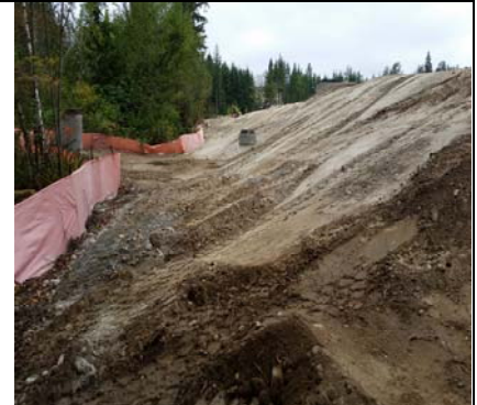
Building The Soccer Field Up
