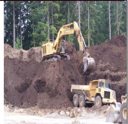
Loading Soil For One More Field Lift
