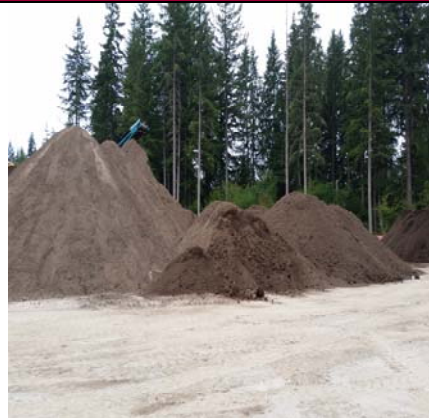
Making Topsoil From Onsite Material
