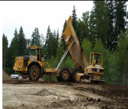
Another Onsite Soil Delivery
