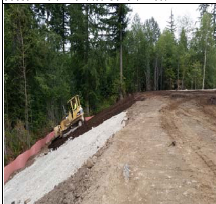
Spreading Soil On The Soccer Field Slopes
