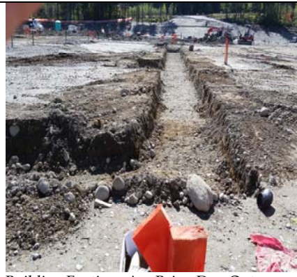
Building Footings Are Being Dug Out
