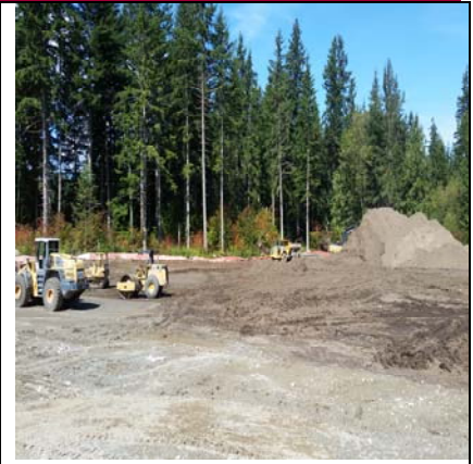
...and The Topsoil Pile Gets Smaller
