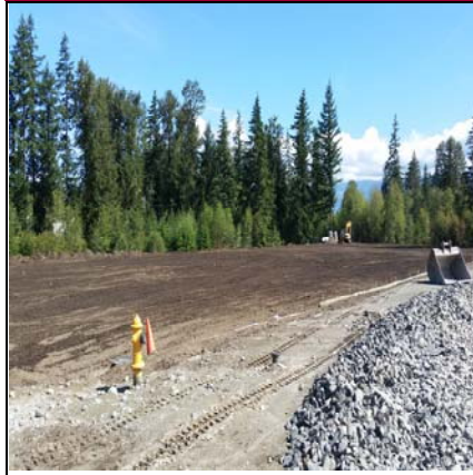
Northeast Field Nearing Completion
