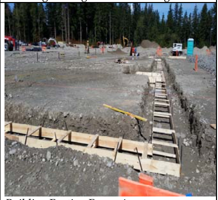
Building Footing Forms 4
