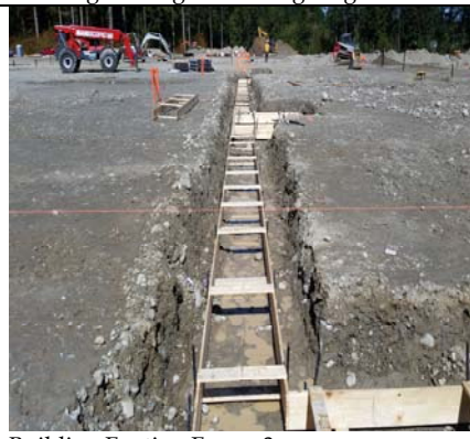
Building Footing Forms 3
