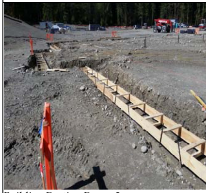
Building Footing Forms 2
