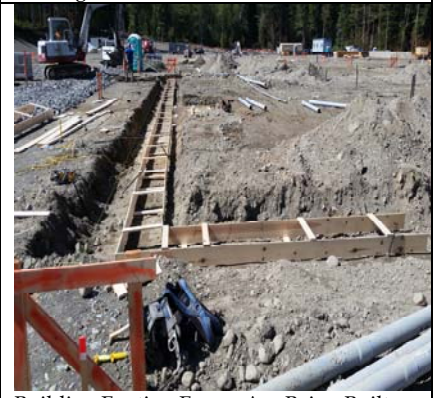
Building Footing Forms Are Being Built
