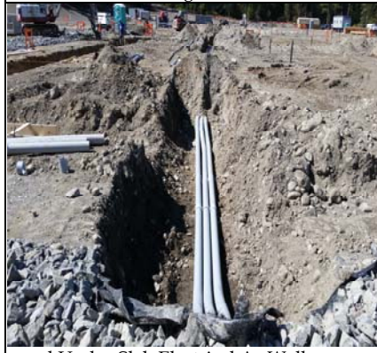
...and Under-Slab Electrical As Well
