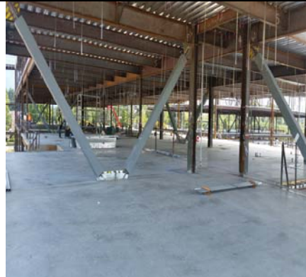
2nd Floor Wall Layout Begins-Area A
