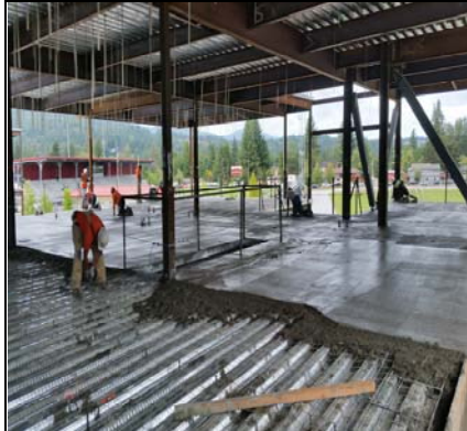
First Slab Concrete Pour-2nd Floor-Area A
