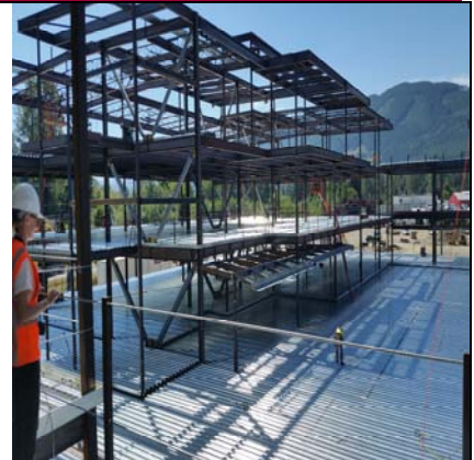
Area B - SE Building Frame & Decking
