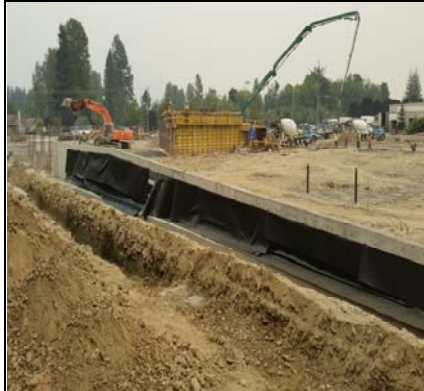
Waterproofing & Forming Retaining Walls
