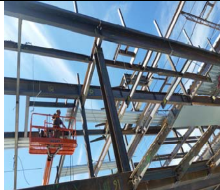
Framing & Decking Area B Connector Building
