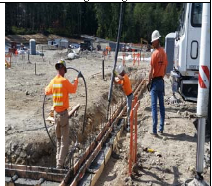
Vibrating The Concrete For A Good Finish
