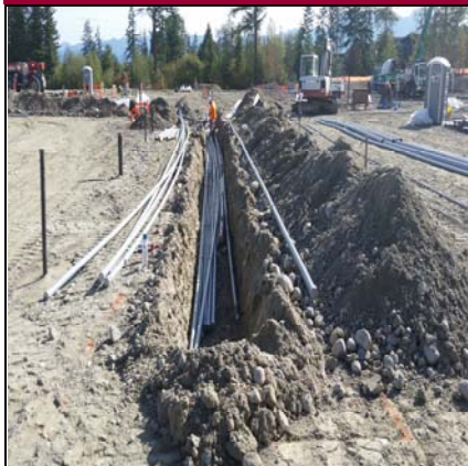
More Underground Electrical/Data Runs
