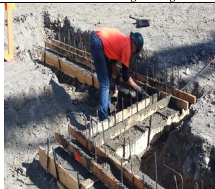
Hand Finishing The Base Top Of Footing
