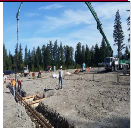
The First Building Footings Concrete
