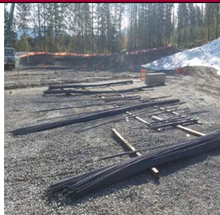
More Steel For The Building Footings
