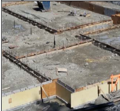
Interior Footings Being Built
