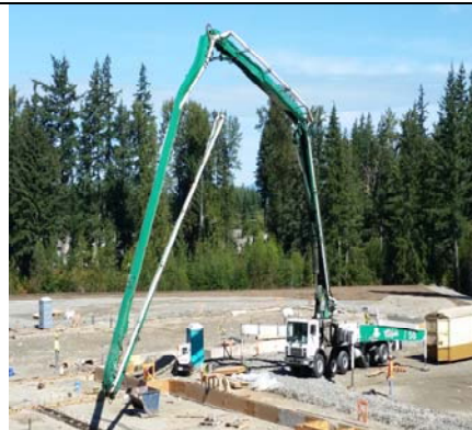
Concrete Pump Truck Set Up
