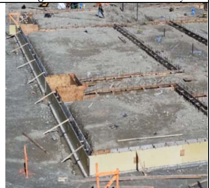
Stem Wall Forms Being Built
