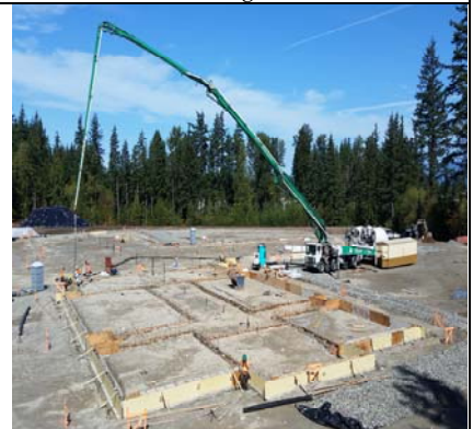
South Classroom Wing Stem Wall Set Up
