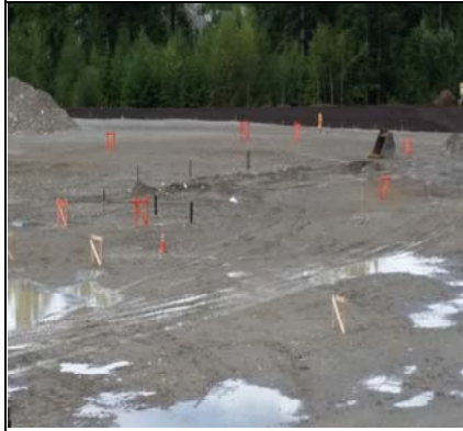
Batter Boards For Building Layout
