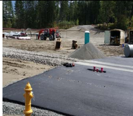
Rock Road Installation For Building Access
