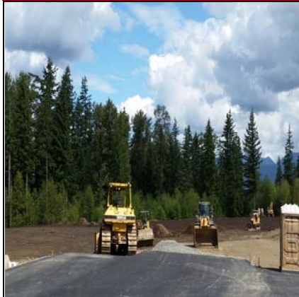
Field Work Shit Down Due To Rains
